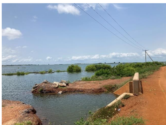
Figure 6-91 - Low Tension Power Line
