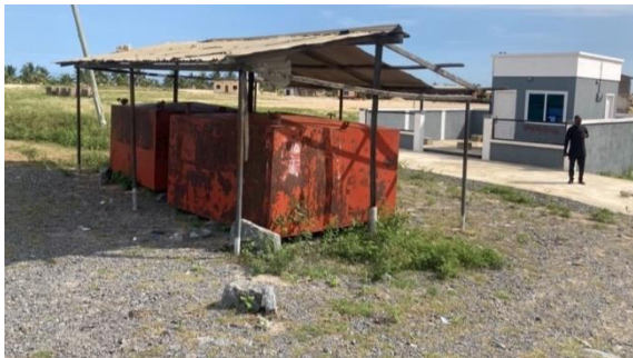
Figure 7-21 - Premix Fuel Station Marked Out by Lands Commission within Designated Area
