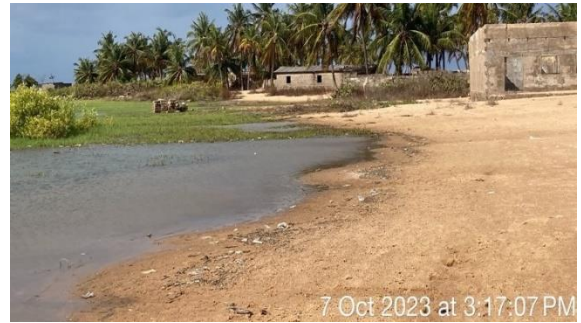
Figure 7-20 - Homes Impacted by Sea Erosion and Lagoon Floods
